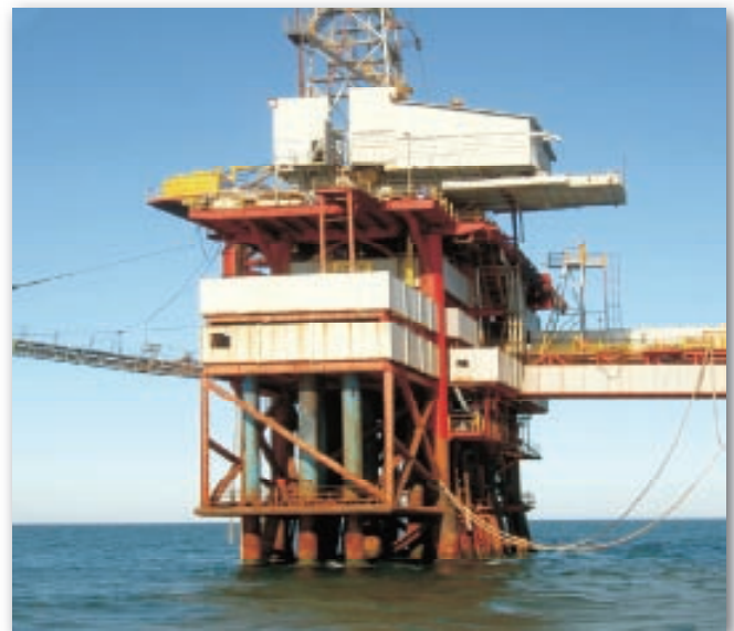
Fig 1- Complex 3D Reality of a site location
